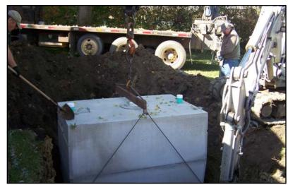
The top of a septic tank had collapsed in at this single family home. The old tank was removed and a new 1000 gallon tank was installed in the same location. 1000 gallons is the minimum size septic tank tank allowed in the county.
